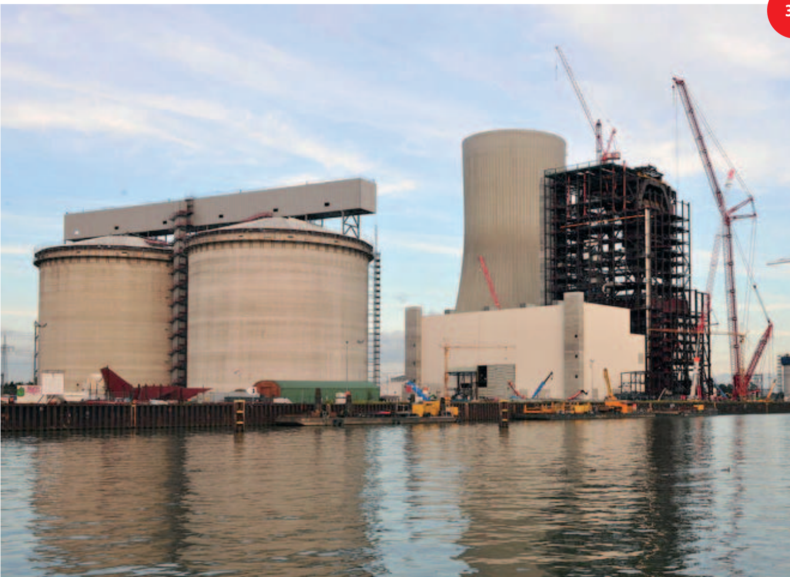
2 x 100,000 m 3 coal silos under construction
