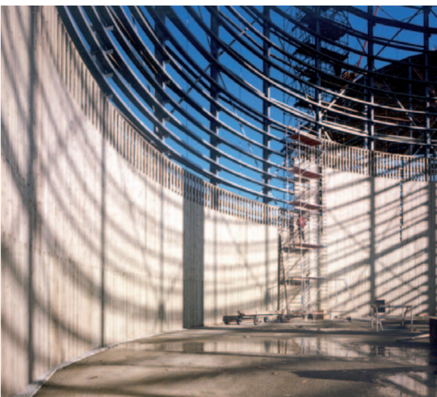
Ammonium sulphate silo with wooden inner wall
