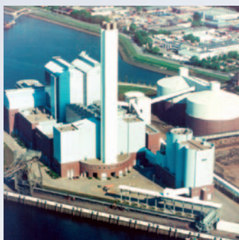
Coal silos and FGD gypsum silo, Germany
